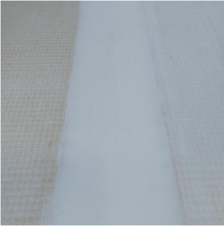
Finished joint prior to painting
